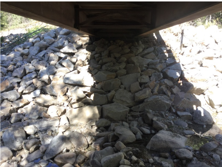
Right Bank Abutment when facing downstream
