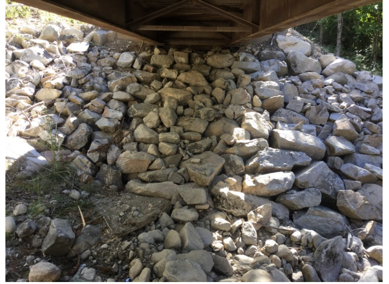
Left Bank Abutment when facing downstream
